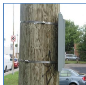
Figure 16, Profile view of pole bracket
