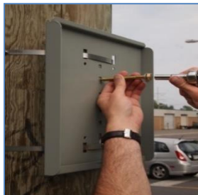
Figure 15, Additional lag bolts should be used for added security
