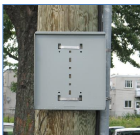
Figure 14, Pole bracket banded to utility pole
